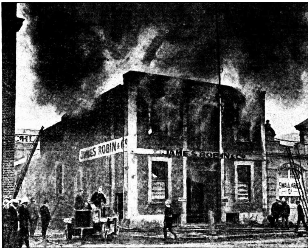
Photos. by H. Krischock. THE MOTOR ENGINE AT WORK.
